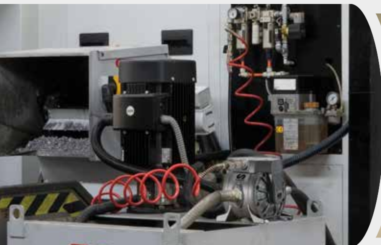
Cutting oil solution transfer.
