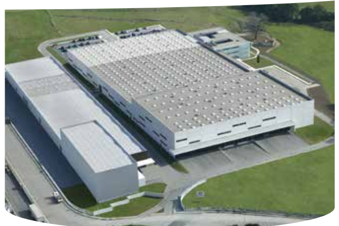
Research & Development and Manufacturing facility in Gijón (Spain)
